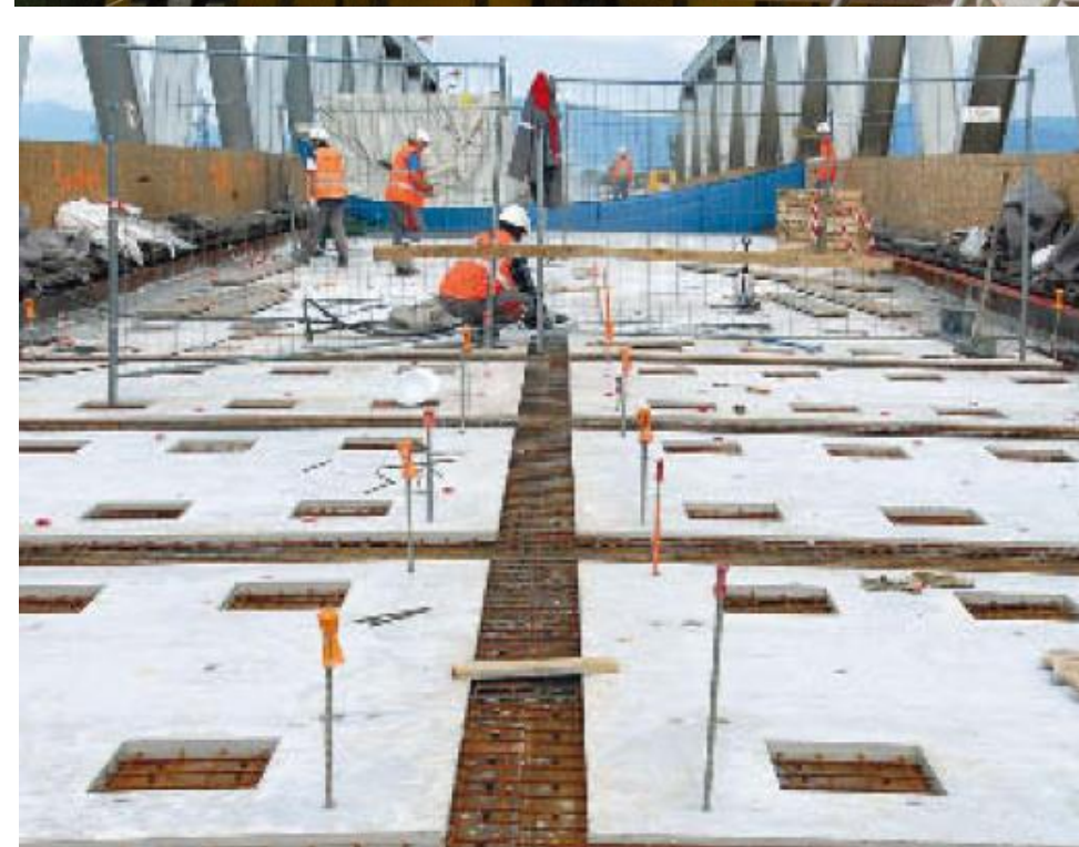
Strengthening of orthotropic steel bridge decks Orthoplus project, 2007-2012 Application on Illzach Bridge, 2011
