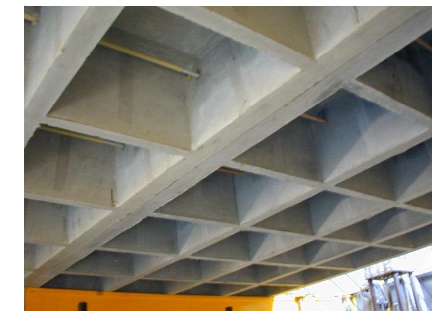
Transversally pretensioned Waffle-slab bridge deck segments Assembled by post-tension MIKTI project, 2003-2008
