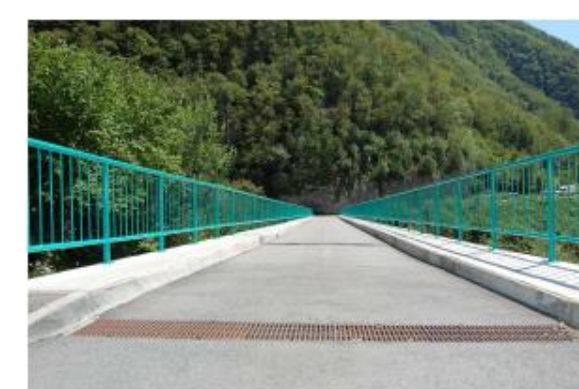
Concrete deck coating using strain-hardening UHPFRC ARCHES project, 2009
